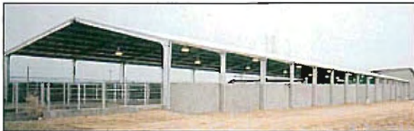
Completed Parlor Barn -- Smith Bros. Dairy, Royal City, WA General Contractor: Mountain States Construction, Sunnyside, WA
