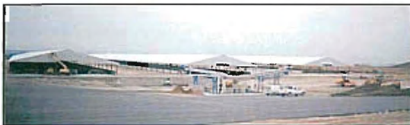
Completed Freestall Barns -- Smith Bros. Dairy, Royal City, WA General Contractor: Mountain States Construction, Sunnyside, WA NOTE Albers Manure Separators in foreground
